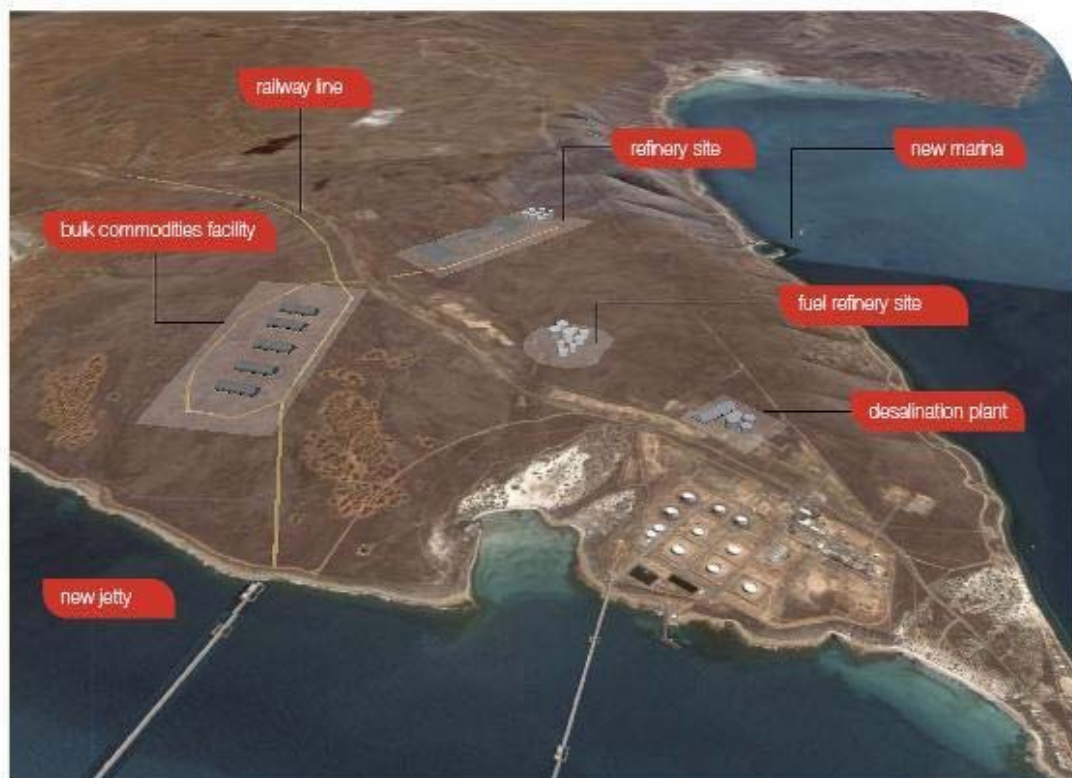
Figure 2 Iron Ore Export Facility at Port Bonython
